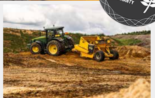
➤ A D8000 leveling the ground of a construction site.
